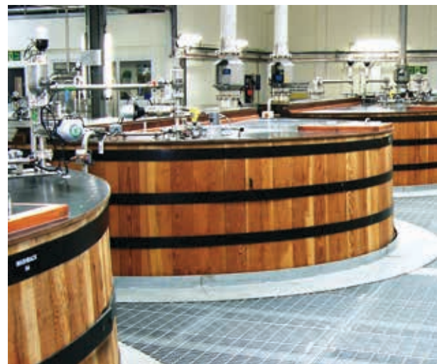
New Douglas fir fermenters at Diageo's Teaninich distillery, Scotland
